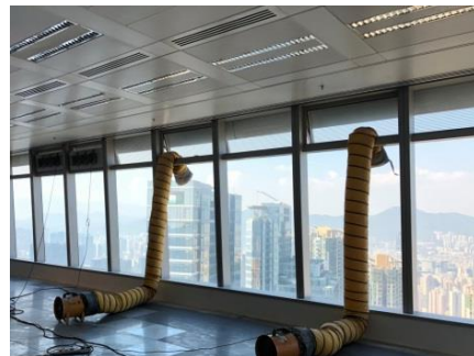
Make use of blowers to enhance air movement during fitting out of premises
