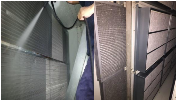
Periodic cleaning of air handling units
